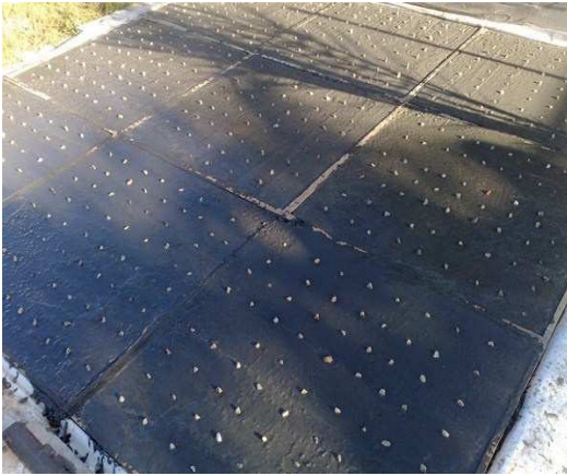
Figure A.5 Finishing fixed aggregates on the first layers surface.
