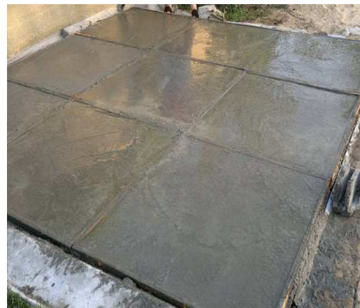
Figure A.12: Finishing the slab surface for second layers.
