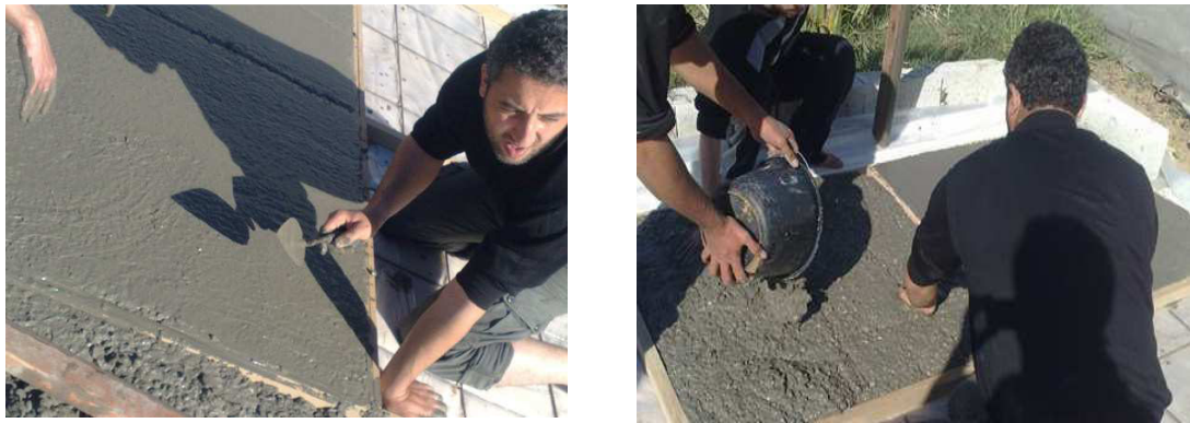
Figure A.2: Filling the template with concrete for first layer slabs.
