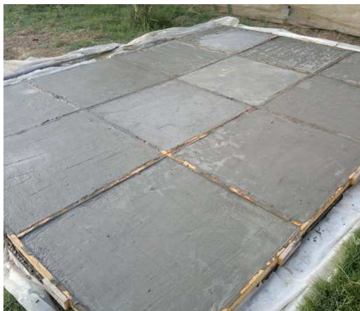
Figure A.12: Finishing the slab surface for second layers.
