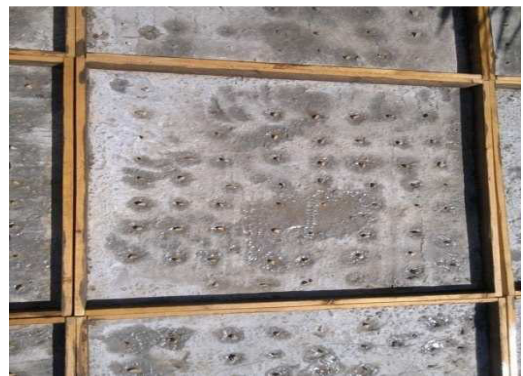
Figure A.6: Preparing the 6 cm template for second layers.
