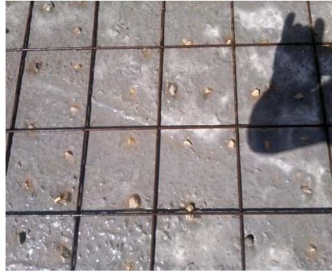
Figure A.7: Preparing the 6 cm template with steel reinforcement for second layers.
