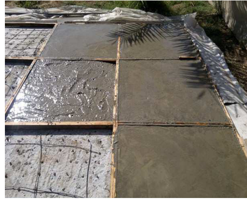
Figure A.10: Filling the second template with concrete for different RLDPE contents.
