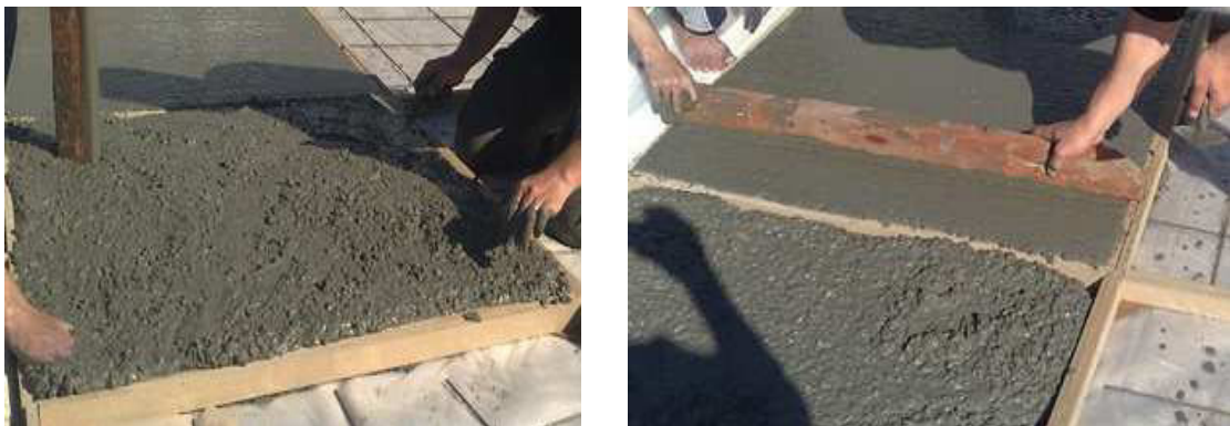
Figure A.3: Finishing the slab surface for first layers.
