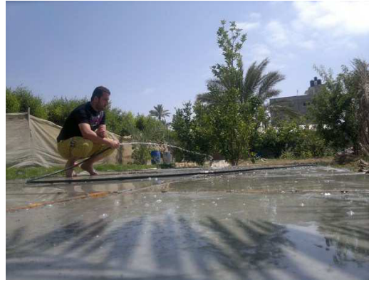
Figure A.13: Curing the second layers.
