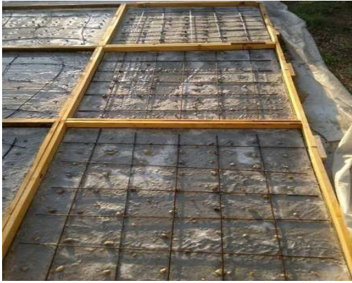
Figure A.7: Preparing the 6 cm template with steel reinforcement for second layers.
