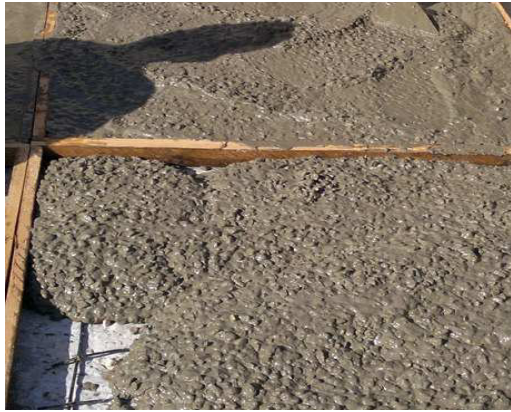
Figure A.10: Filling the second template with concrete for different RLDPE contents.
