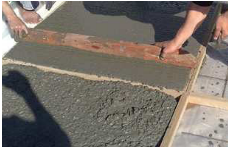
Figure 3-18: Finishing the slab surface for first layers.
