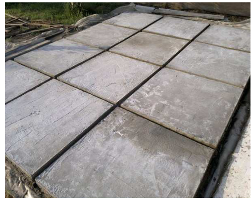
Figure A.14: Slabs after remove the Template
