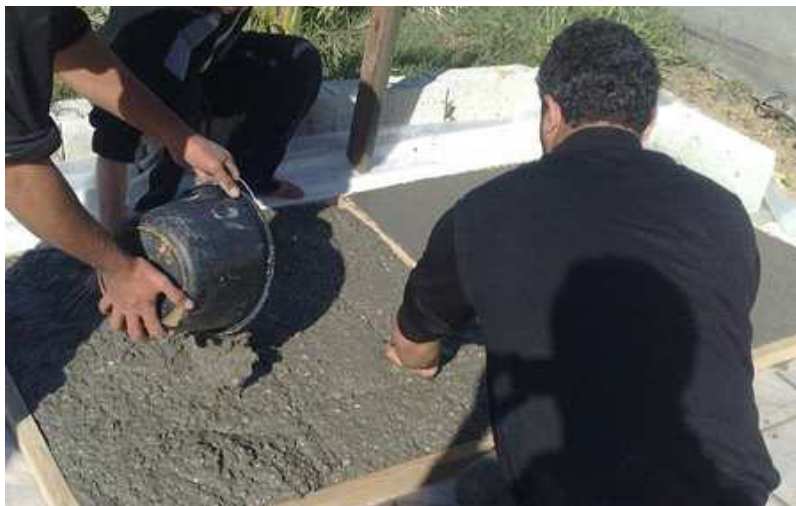
Figure 3-17: Filling the template with concrete for first layer slabs.
