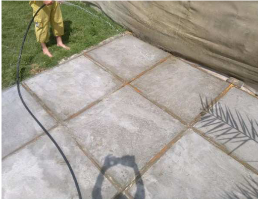
Figure A.13: Curing the second layers.
