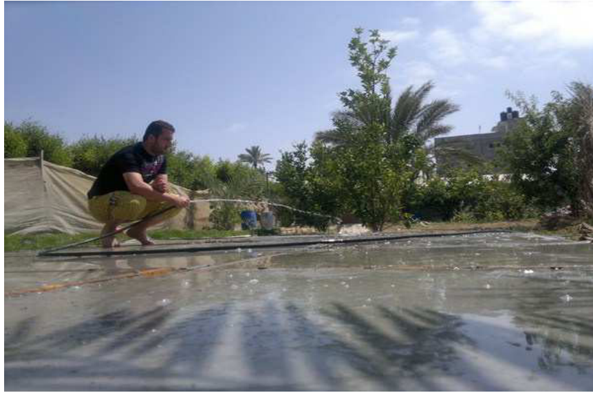
Figure 3-26: Curing the second layers.
