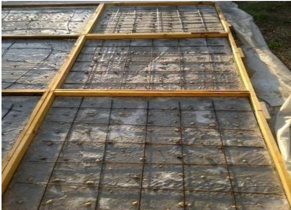
Figure 3-25: Preparing the 6 cm template with steel reinforcement for second layers.
