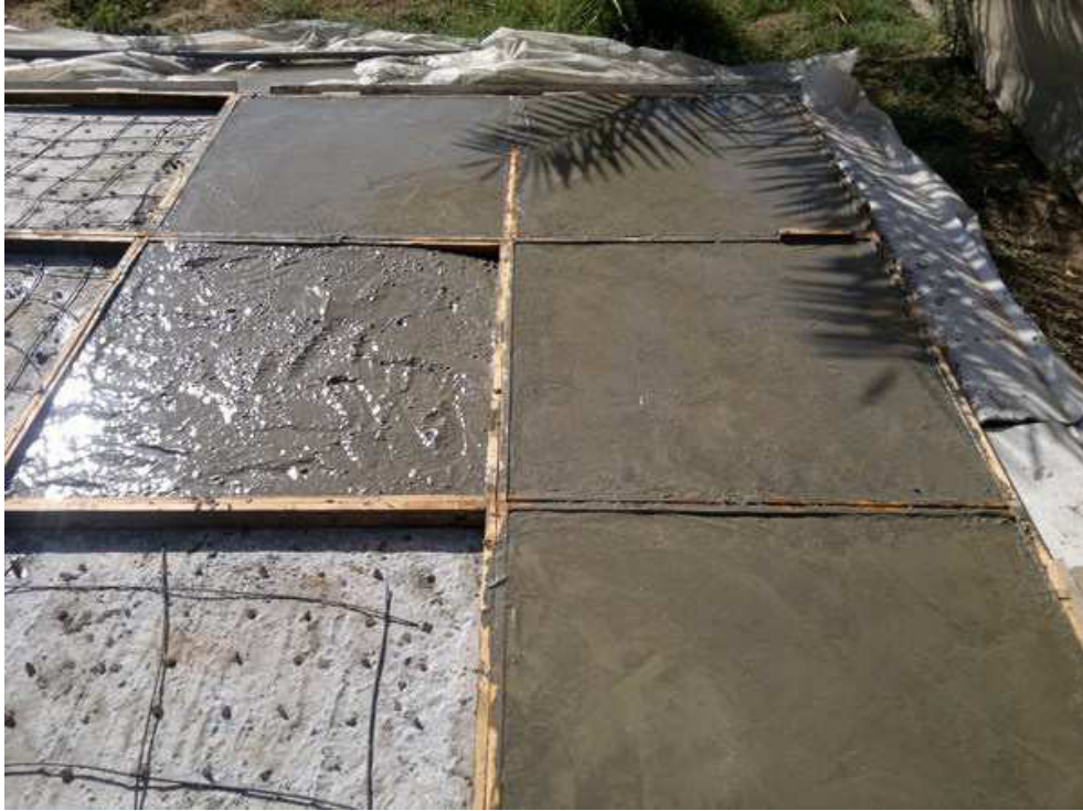
Figure 3-24: Filling the second template with concrete for different RLDPE contents.
