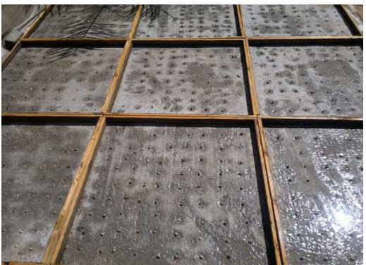
Figure A.6: Preparing the 6 cm template for second layers.
