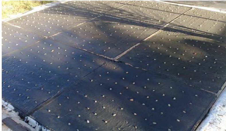
Figure 3-20: Finishing fixed aggregates on the first layers surface.
