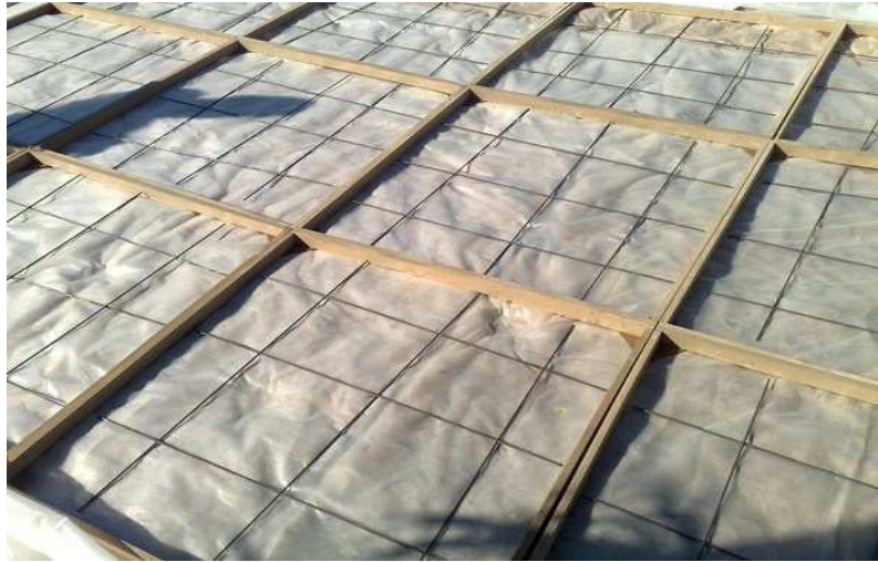
Figure 3-16: Preparing the 4 cm template with steel reinforcement for first layers.
