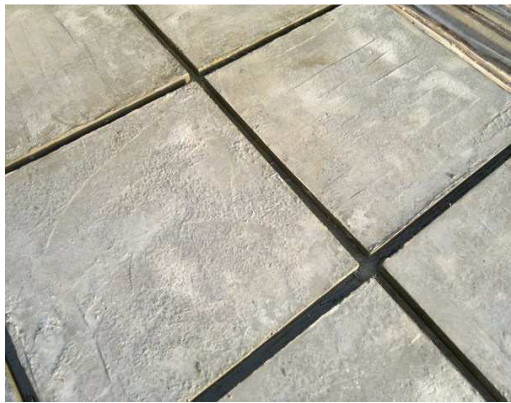
Figure A.14: Slabs after remove the Template
