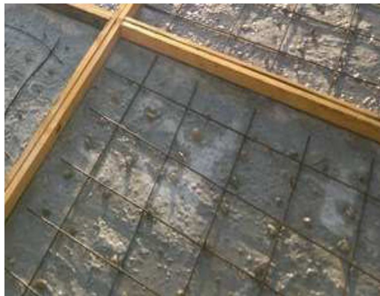
Figure 3-10: Steel secondary reinforcement used in second layer.
