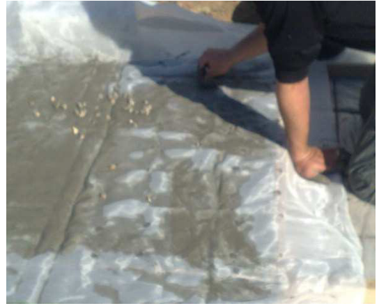
Figure A.4: Fixed aggregates on the first layers surface.
